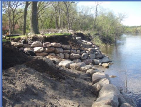
Designs from Houston Engineering specified hard armoring was required to stabilize the toe of the slope. Rip rap was overlaid on geotextile fabric to provide a bank structure that prohibits further erosion.
