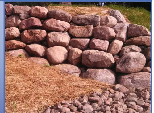
Stabilization mats (on left) with percussion anchors were used to further protect shoreline access around rip rap. A native grass buffer was also planted at the top of the banks to reduce overland erosion.
