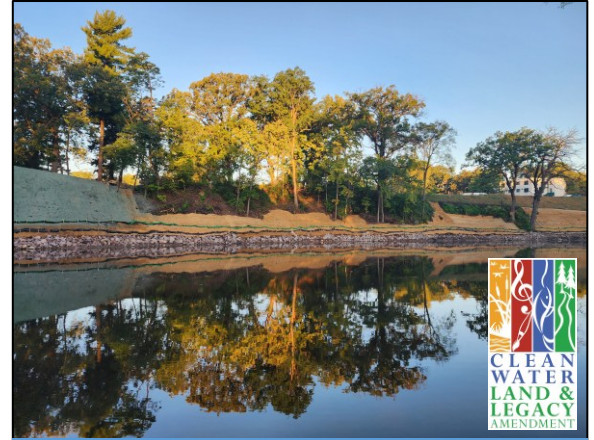
Rum Riverbank Stabilization at the Woodbury House site in Anoka
