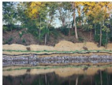
Shoreline protections after construction.
